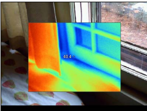
Weatherstrip and caulk windows.
